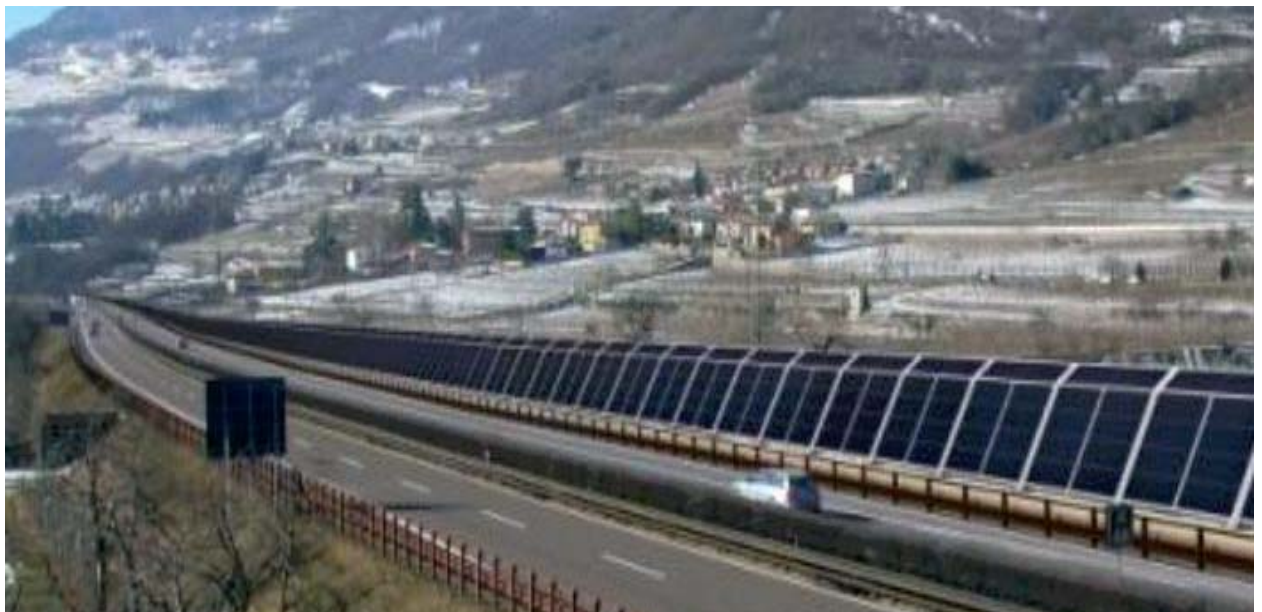
Figure 8.6: In this example, the noise barrier is constructed using solar panels, therefore, playing a dual role in mitigating noise and generating electricity for road use or the grid
