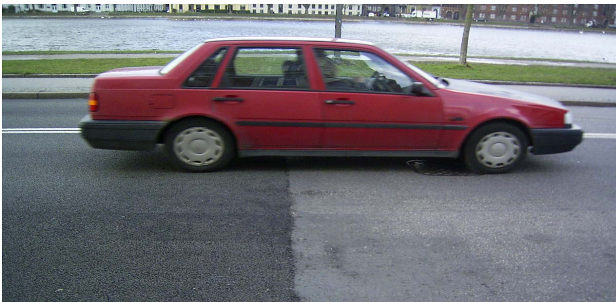
Figure 8.7: An example of a new low-noise surface in Copenhagen: the low-noise surface on the left is 6 dB(A) lower than the dense asphalt on the right [20]
