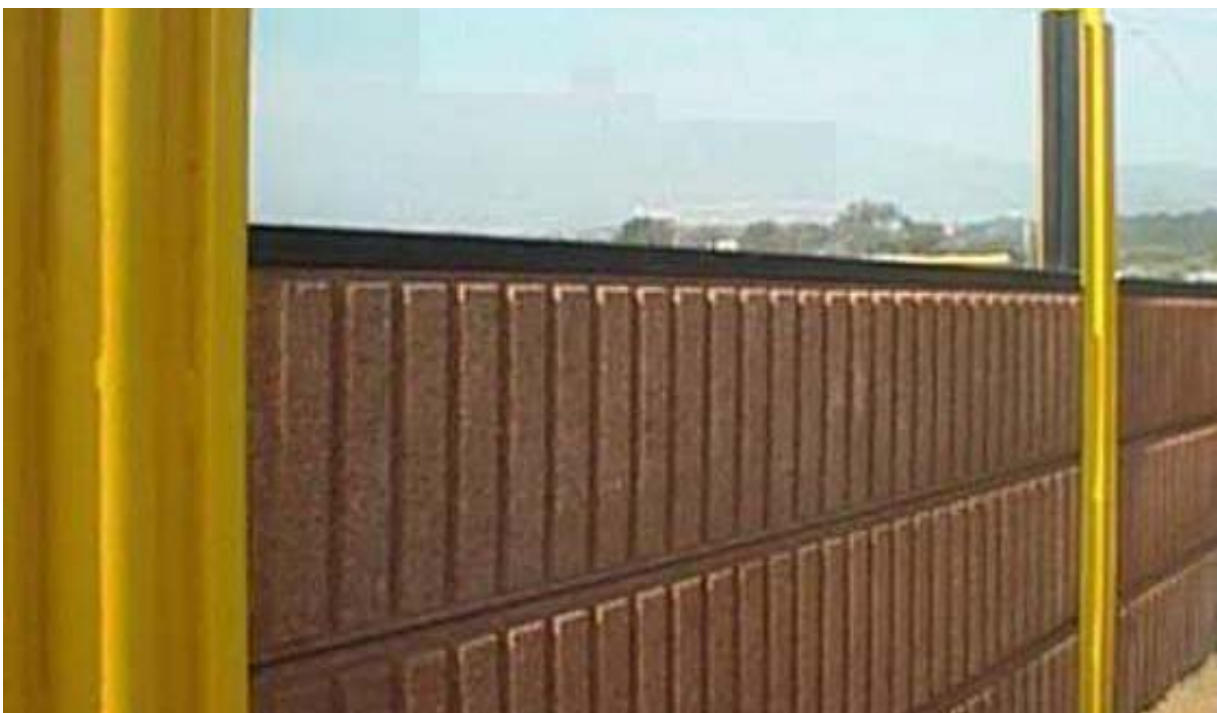
Figure 8.13: A noise barrier made with woodcrete with a transparent section on the top of the barrier. Note the robust support posts. Woodcrete is made from concrete mixed with wood and can be colour rendered to match the environment
