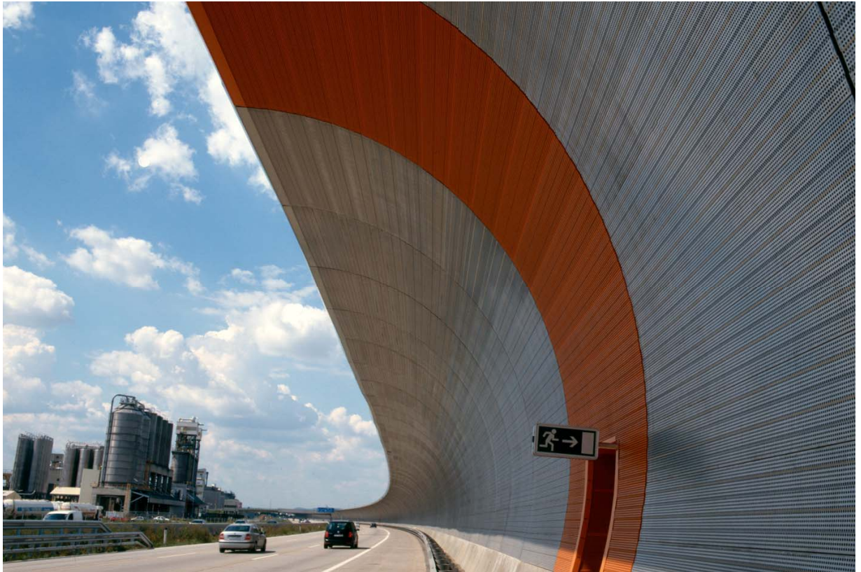
Figure 8.23: Example of a curved noise barrier in Vienna that will affect the propagation of noise
