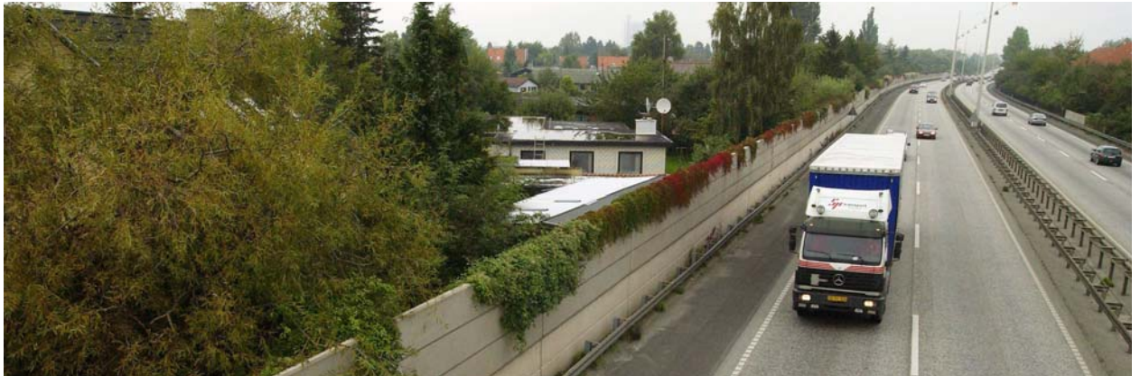
Figure 8.2: An example of a concrete noise barrier. The aesthetic of such barriers can be improved by promoting the growth of vegetation over the top of the barrier, however, this may have implications for the ability of the barrier to mitigate noise.
