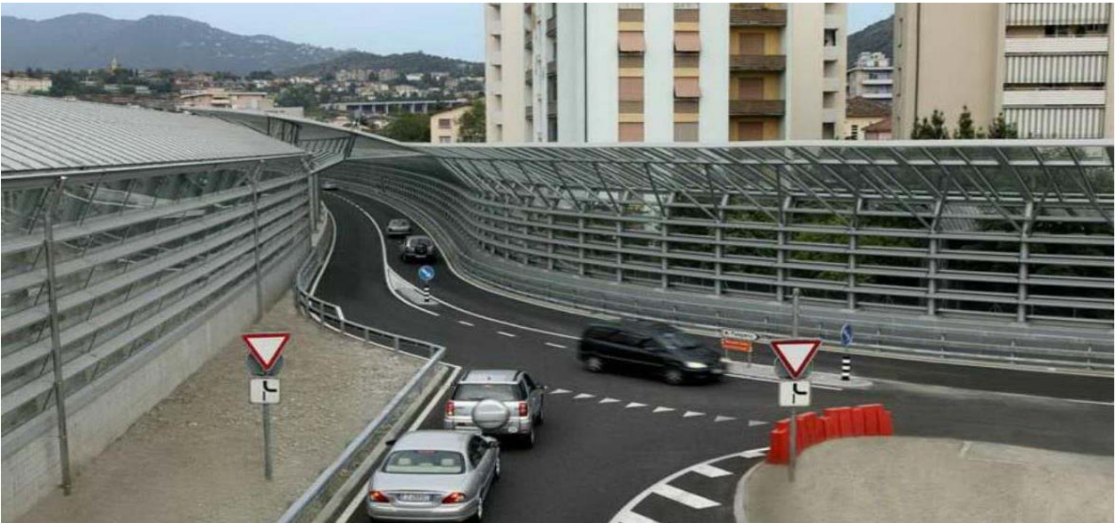
Figure 8.3: Sophisticated arrangement of noise barriers in an urban setting in Italy
