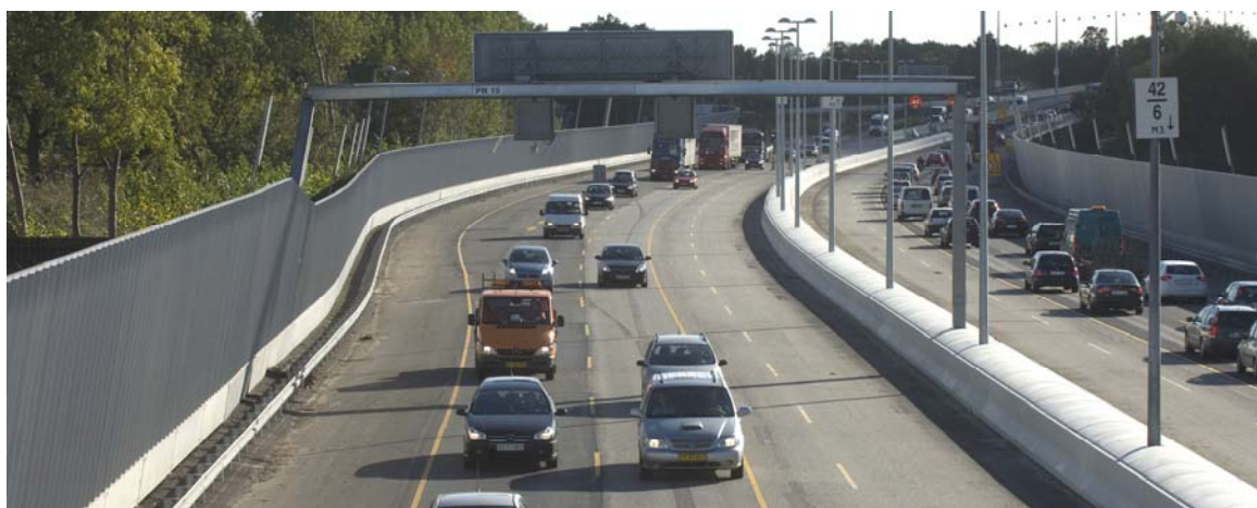
Figure 4.1: The ring road around Copenhagen in Denmark is being widened from four to six lanes through a densely built-up residential district. In order to reduce noise, noise-reducing thin layer pavements and 4-m high noise barriers are included in this large road reconstruction project.
