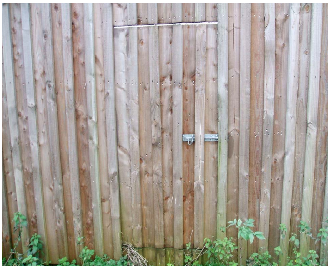
Figure 8.16: Example of a timber noise barrier showing a poorly fitted access door; note the opening over the top of the door
