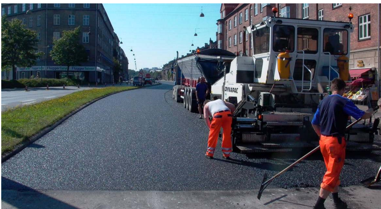
Figure 7.1: The type of pavement used has an influence on the tyre/road noise level on a given road. Here, a noise-reducing two layer porous pavement is applied on top of an existing main road in Copenhagen, Denmark, as a part of the ongoing road maintenance process.
