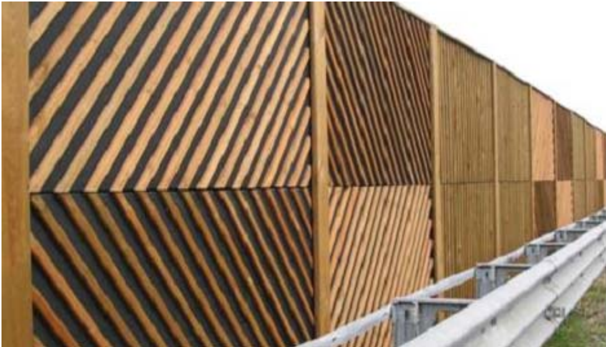
Figure 8.12: An example of a timber noise barrier
