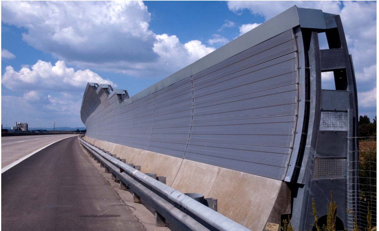
Figure 8.27: Example of a curved noise barrier with staggered height; barrier dimensions may vary depending according to the location
