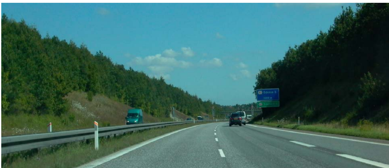
Figure 8.1: A vegetative earth berm acting as a noise barrier in Denmark
