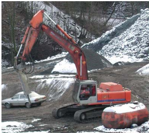
Figure 9.1: An example of a noisy activity: use of spike hammer (photo: Norwegian pollution control authority)
