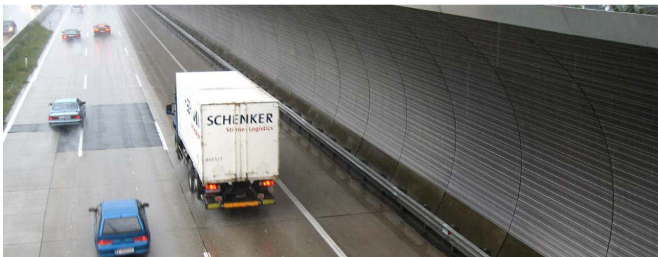
Figure 4.4: The highway from Vienna to the international airport has been widened with extra lanes. On a long section, the highway passes a residential area. In order to reduce the noise a 5.5 m high noise barrier in a curved shape bending over the road has been constructed.
