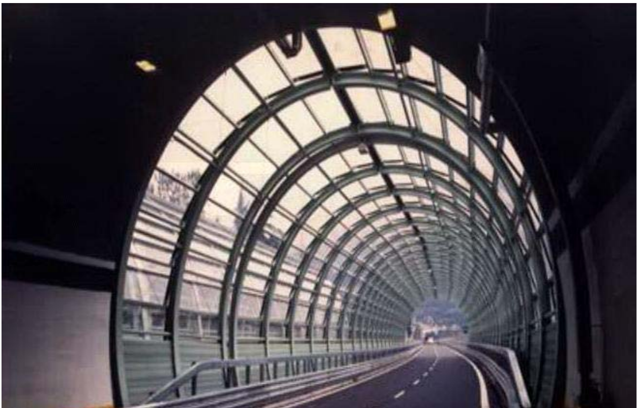
Figure 8.26: Example of a road completely enclosed for noise reduction purposes
