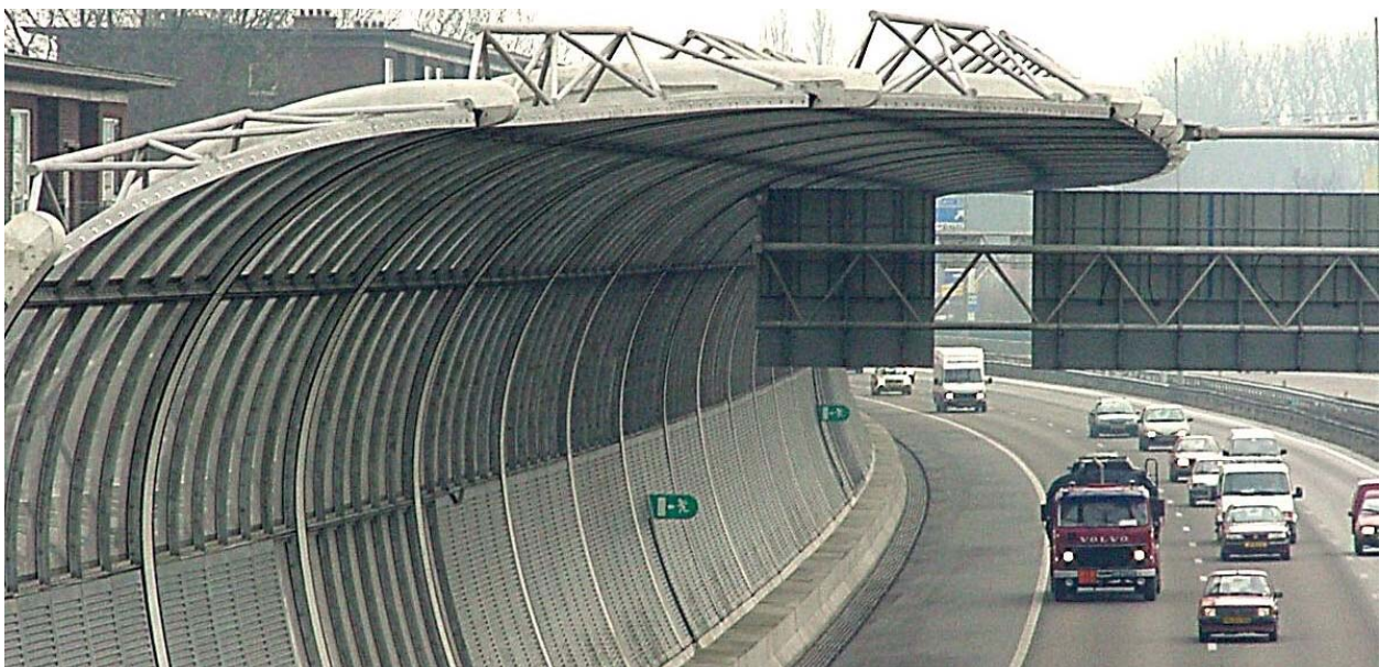
Figure 8.24: Another example of a curved noise barrier in the Netherlands, in this case, partially enclosing the road. Barriers may be designed to provide additional mitigation in areas with sensitive receptors nearby.
