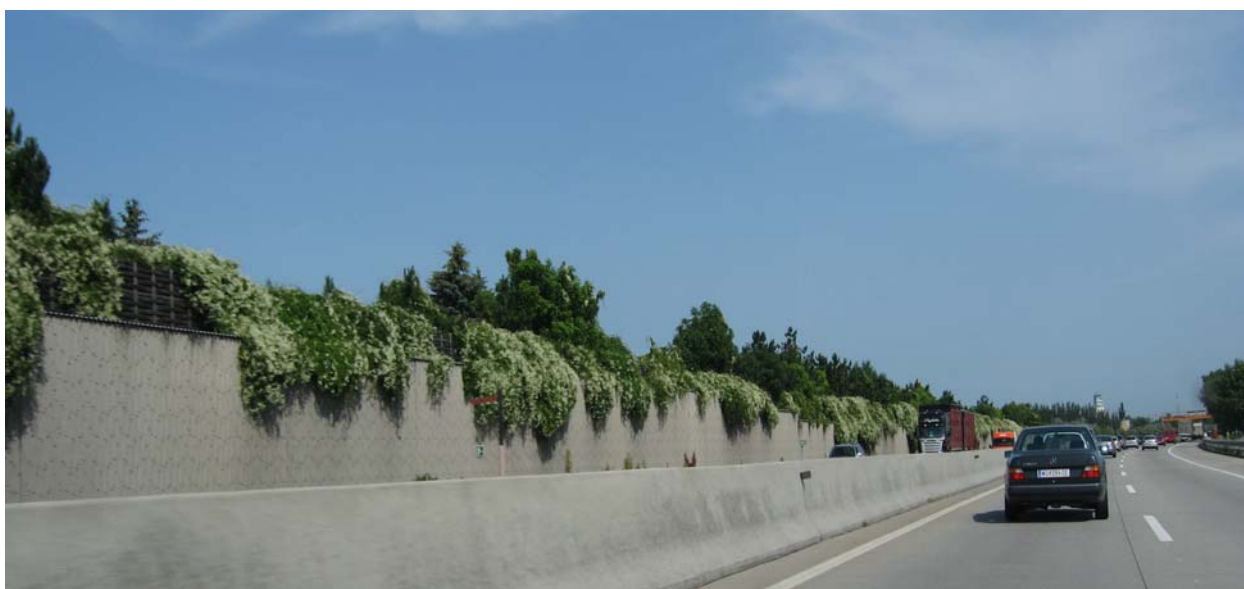
Figure 8.11: An example of a concrete noise barrier with vegetation growing over the top of the barrier. The vegetation on the top of the barrier may have the potential to impact on its acoustic properties.
