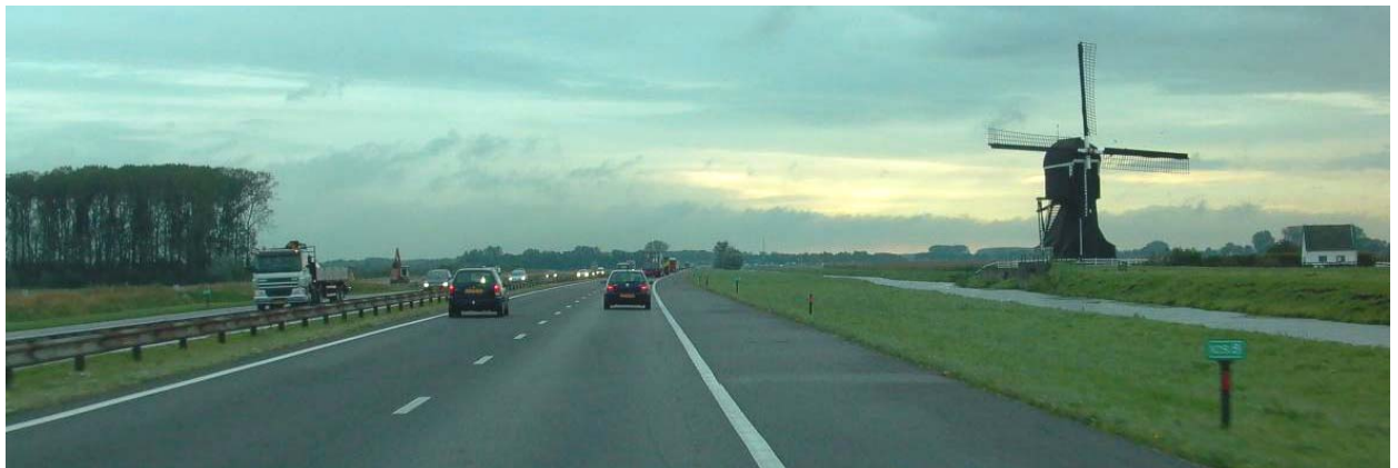
Figure 7.2: In the Netherlands, the use of porous asphalt on highways is a national policy guideline. In 2008, around 80% of the network featured porous asphalt
