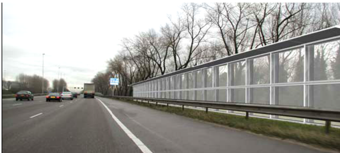
Figure 8.22: Example of T-top noise barrier design used in the Netherlands
