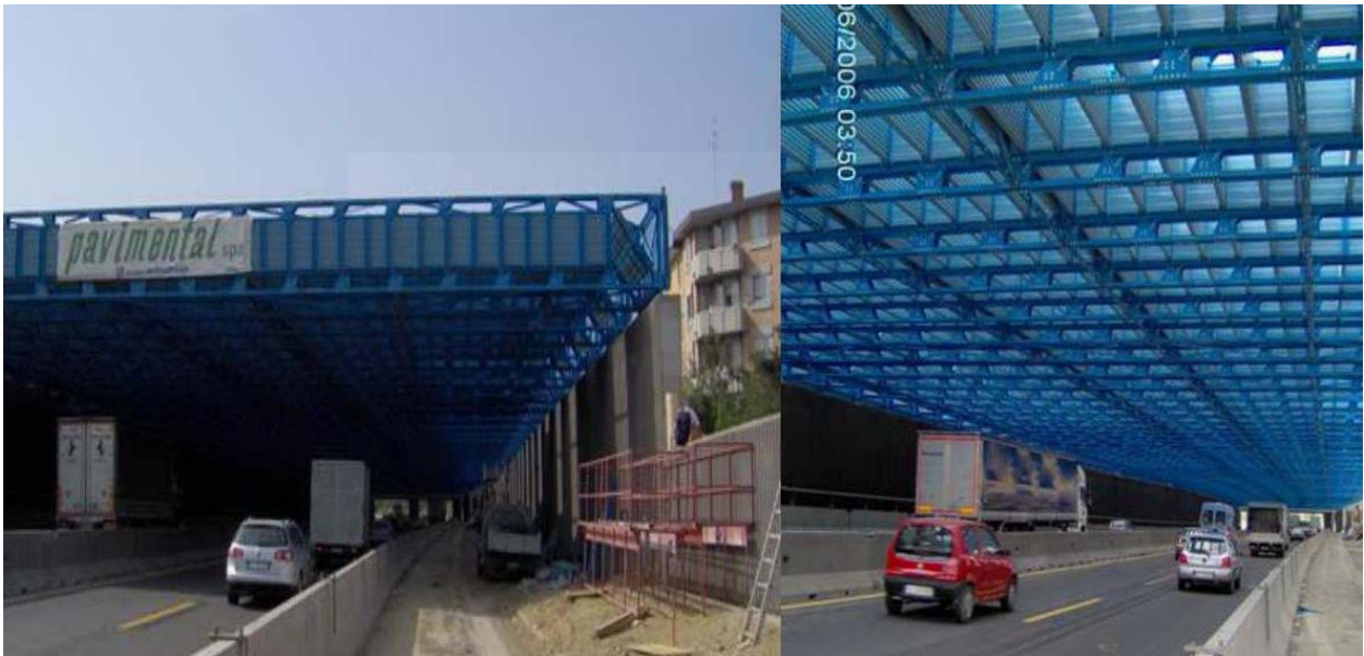
Figure 8.25: Example of a partially enclosed road in Italy with a noise barrier constructed overhead; note the vertical alignment of the barriers overhead
