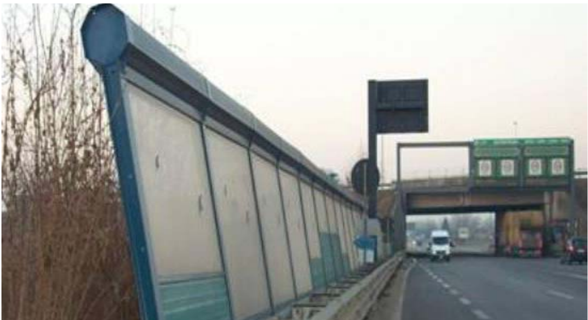
Figure 8.20: Example of a variation of the T-top design; this example shows a barrier with an octagonal top
