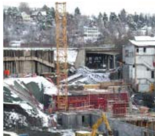
Figure 9.2: Construction activity in a densely built-up area (photo: Norwegian pollution control authority)
