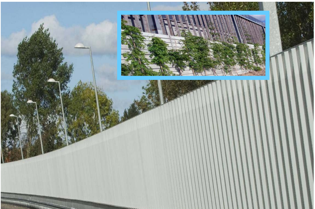
Figure 10.2: New noise barrier constructed as part of the modifications to the Motorring 3 in Copenhagen, Denmark
