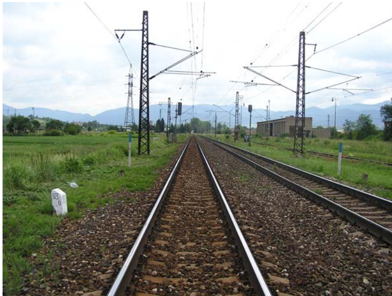
Figure 5: Position for measurements at straight railway track
